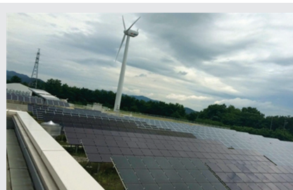
Wind Power Generation at the Fukushima Renewable Energy Institute
